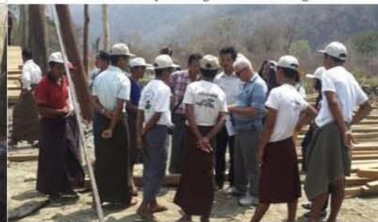
On-Job Training at Construction Site
