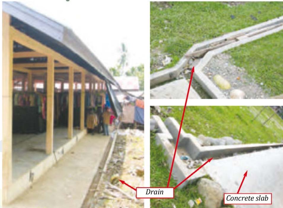
Well built ditch around the slabs of the sheds
