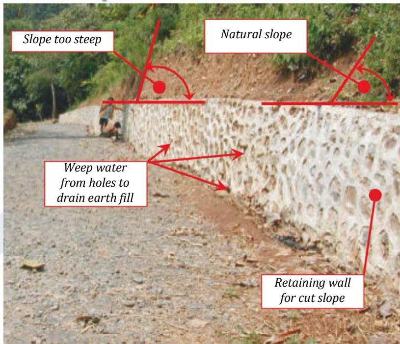
Retaining wall for cut slope
