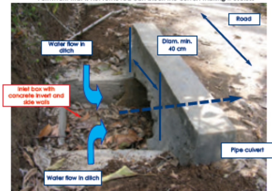
Inlet box for a pipe culvert
