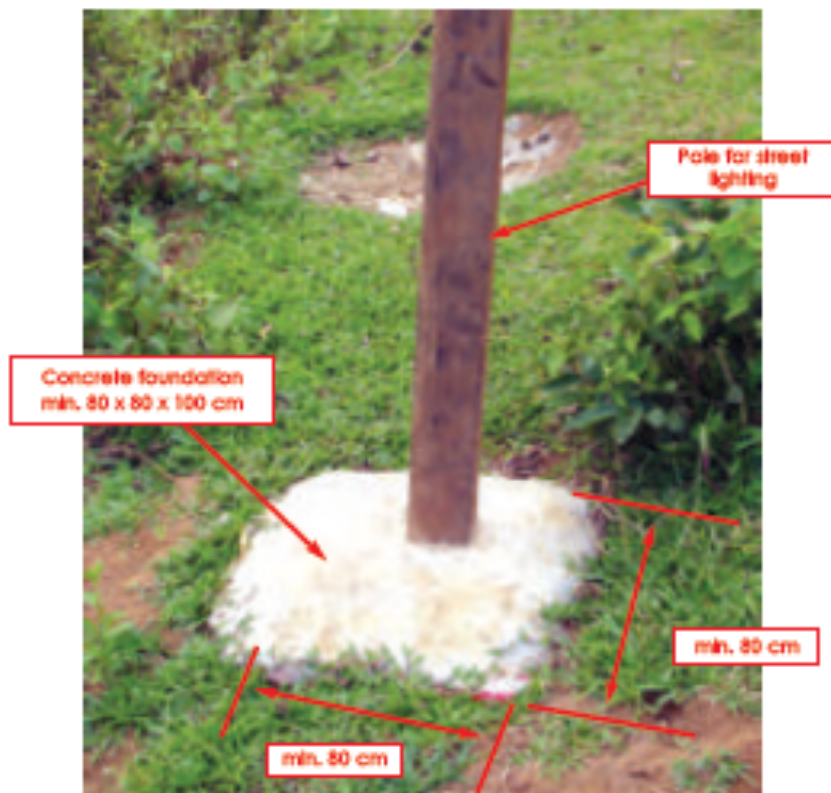
Foundation for a street lighting pole
