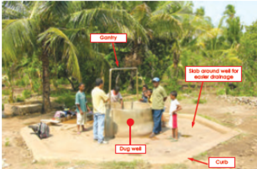
Dug well with all necessary facilities
