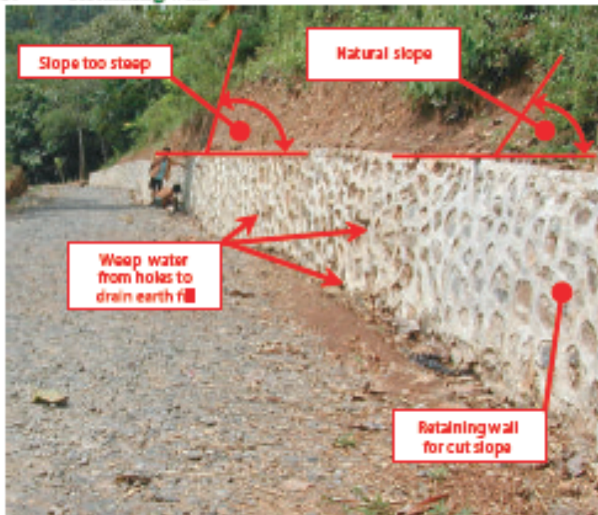
Retaining wall for cut slope
