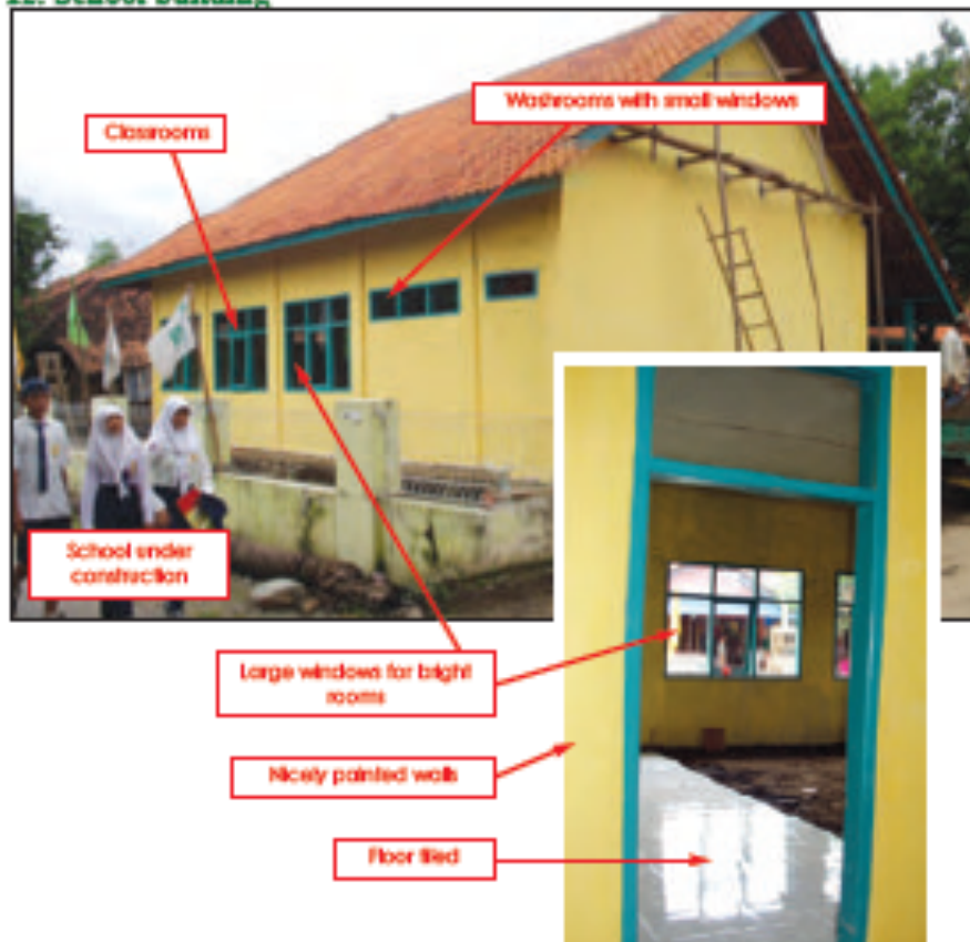
Well-built school building
