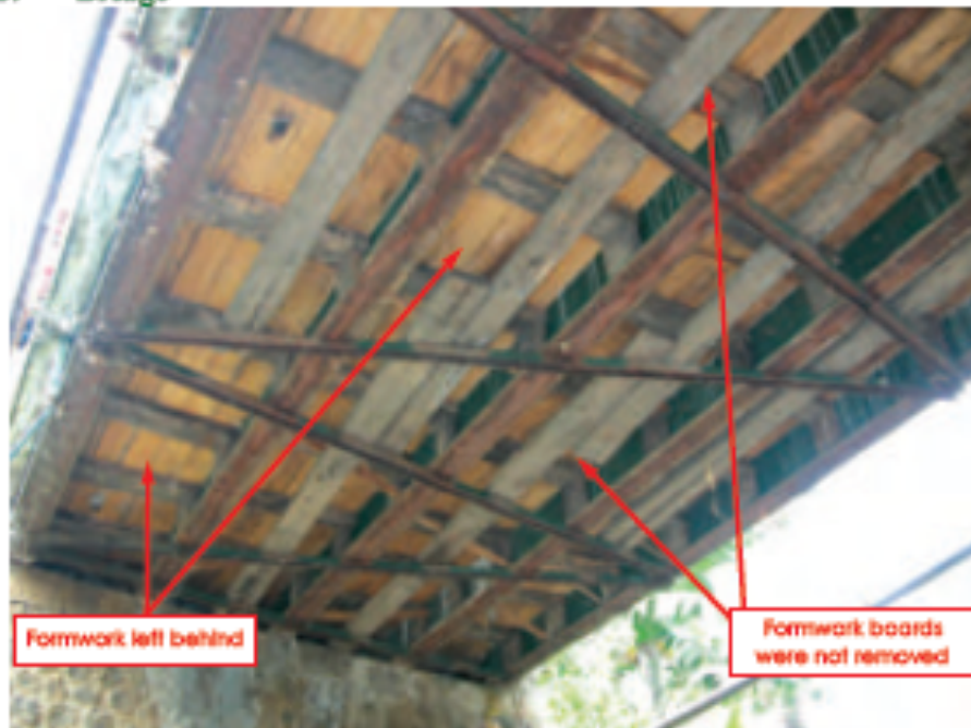
Formwork from under the concrete slab must be removed
