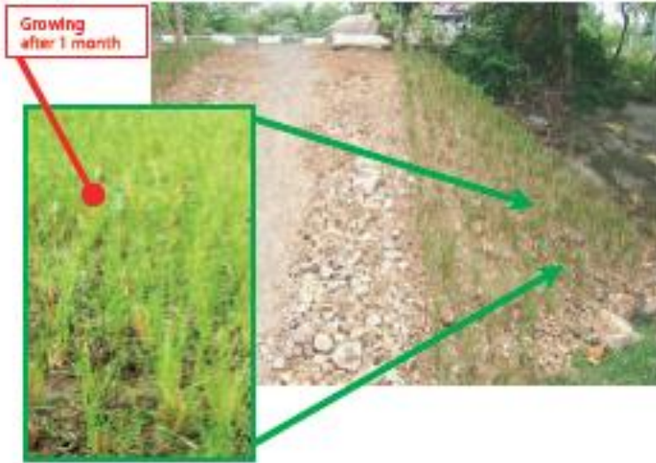
Fast-growing grass was planted on cut and embankment slopes of this road
