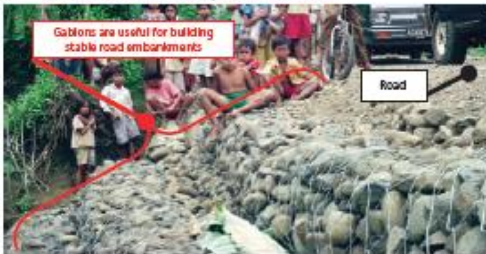
Gabions are used to build a stable embankment slope
