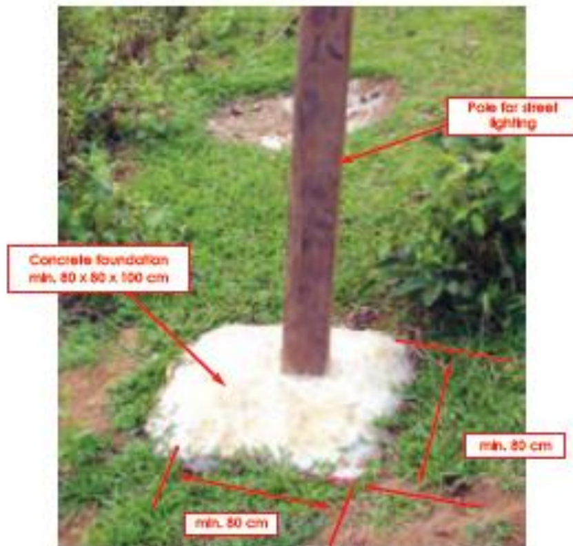
Foundation for a street lighting pole
