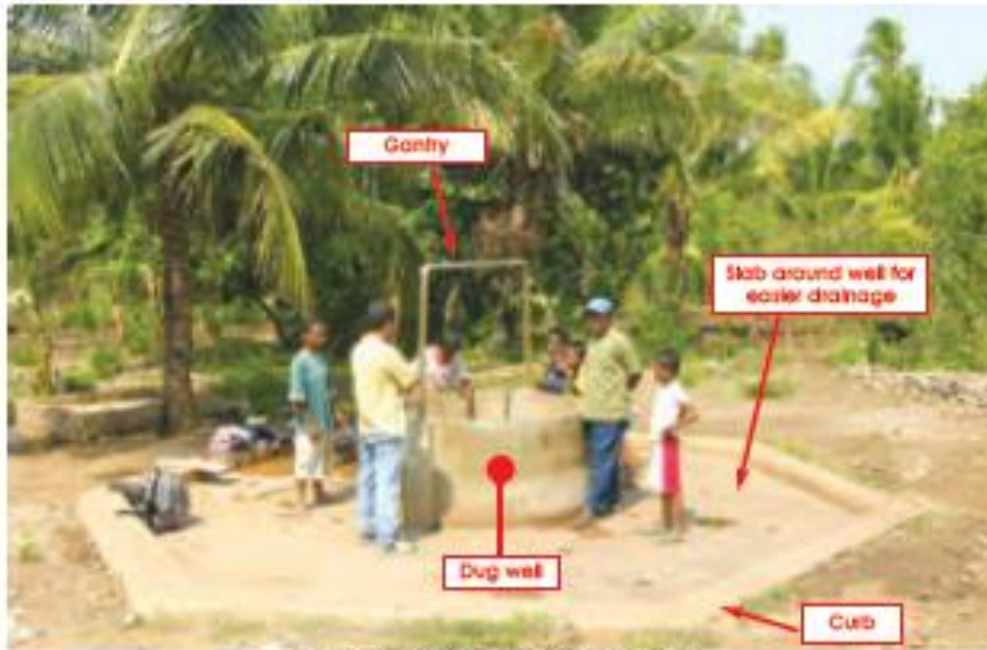
Dug well with all necessary facilities
