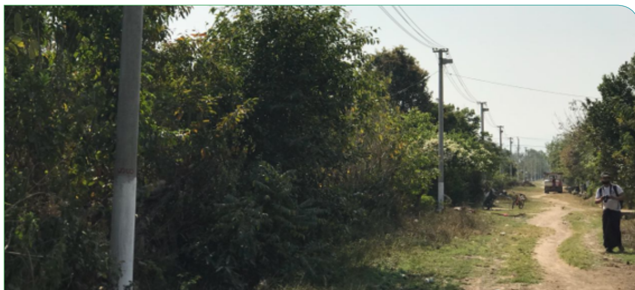
Note: Proper clearance of vegetation from electrical alignment, Bar Do village, Daw Paw Ka Le VT, Loikaw township.
