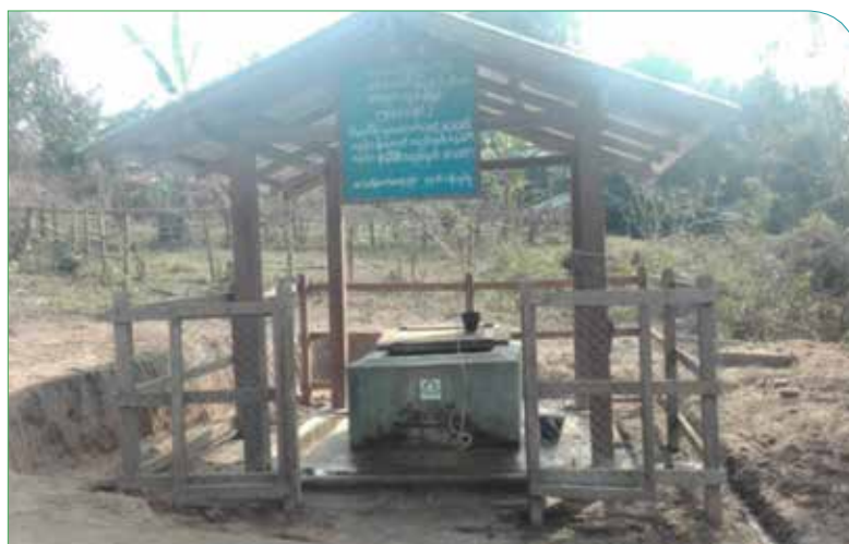
Note: Good example of proper fencing around water supply well, drainage ditch, shelter. Whay Man Kaw village, Naung Kan VT, Banmauk township.
