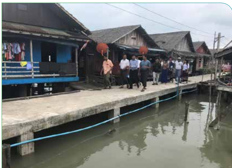
Note: Concrete jetty/pedestrian access, Panzin village, Taw Pyar VT, Kyunsu township.
