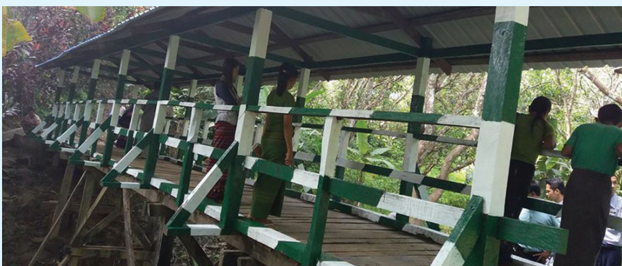
Bridge renovation (After)
