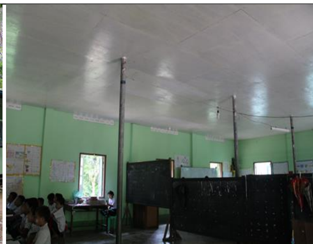
The School Head Mistress pointed out the lighting issues in this room, for low area window openings,
