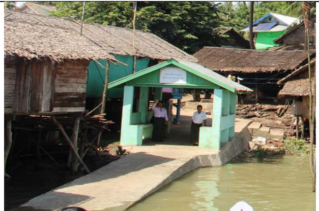
Lin Malo village Jetty approach road
