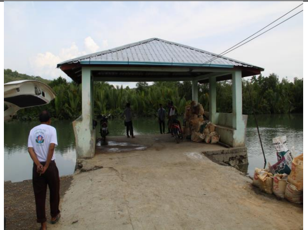
Kattalu Village Jetty construction (Most of the Car for Kyun Su villages can loaded from this Jetty) observed the structure is strong enough,
