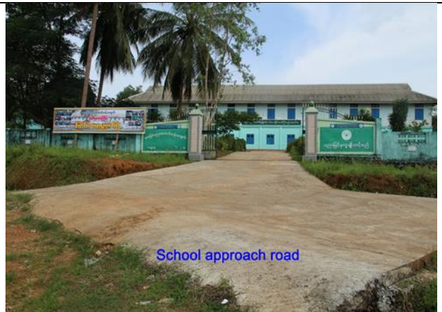
Village roadway is working well, good quality,
