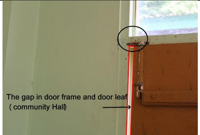
The doorway quality due to un seasoned timber used (gap between door frame and door leaf)
