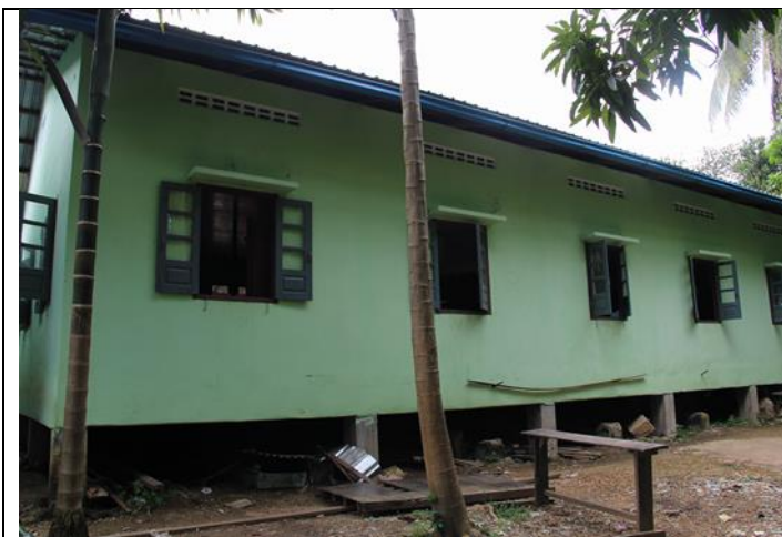
Pa Htaw Village, school construction, RC frame and pucca structure,
