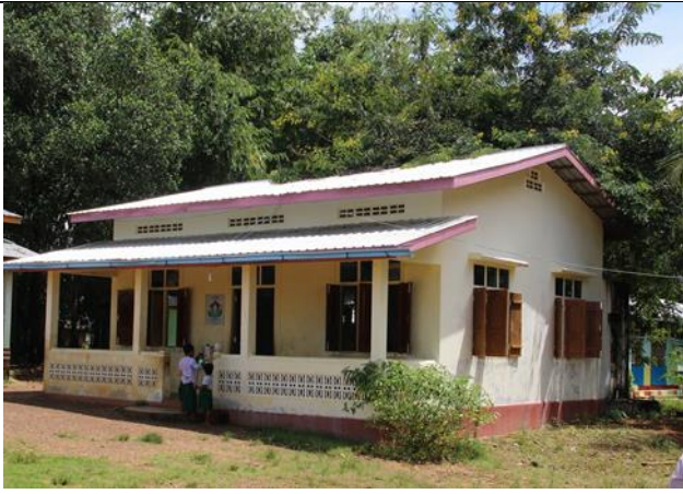
Lin Malo village Primary School construction
