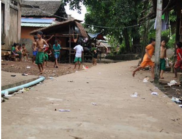
Ma San Par Village, Village road need shoulder strengthening, to be sustainability,
