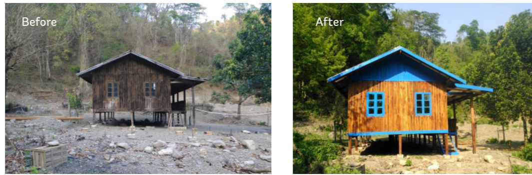
School Renovation Subproject | Yan Se Village, Kanpetlet Township, Chin State
