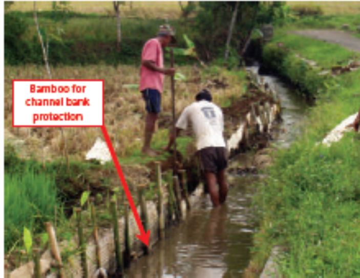
Bamboo stakes and slats can also be used for bank protection on small streams or irrigation channels
