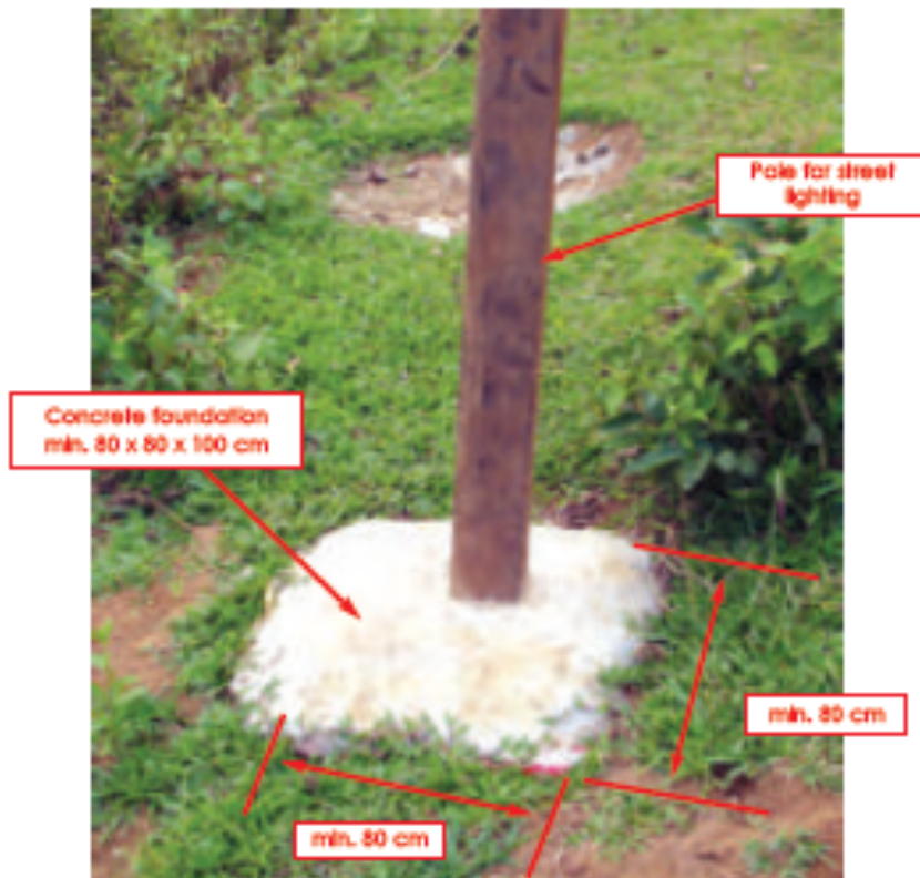
Foundation for a street lighting pole
