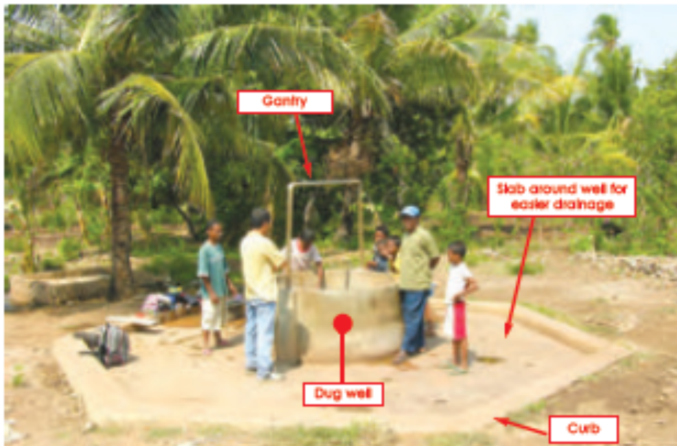
Dug well with all necessary facilities
