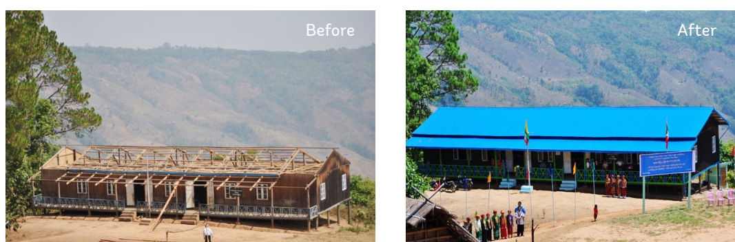
School Renovation Subproject | Par Kon Village, Kanpetlet Township, Chin State
