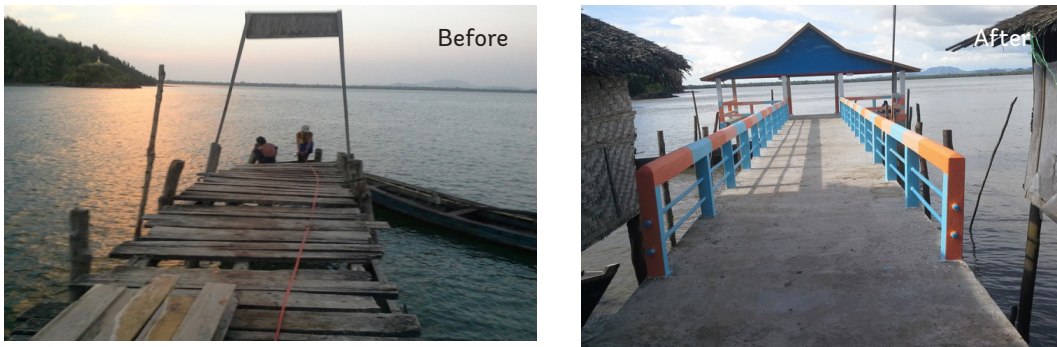
Jetty Subproject | Kawka Hnin Village, Kyunsu Township, Tanintharyi Region
